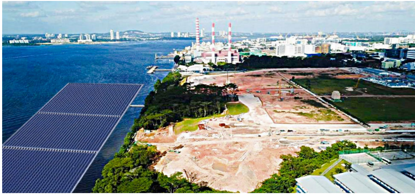
Located along the Straits of Johor, Sunseap's 5 MWp solar farm is one of the largest offshore floating system in the world. The amount of solar energy generated will reduce greenhouse gas emissions by about 2,600 tonnes a year.
