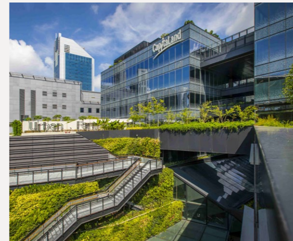
Funan, an integrated development in Singapore developed by CapitaLand Group, boasts the largest area for urban agriculture in the city with a 1,672 m 2 food garden, and a 464 m 2 urban farm located within it.
