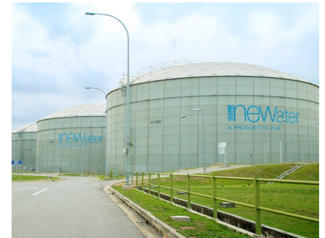
Singapore's first NEWater plant, which is located in Bedok, began operations in 2002.
