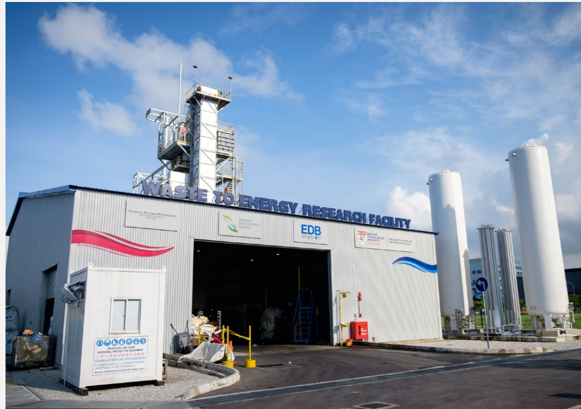
The NTU WTERF is equipped to undertake waste-to-energy and waste-to-resource processes and able to produce syngas to power the plant and slag that can be used for construction.
