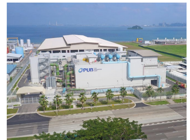
The Tuas Desalination Plant is the first in Singapore to be fitted with solar panels, with more than half of the total roof area covered by solar panels. The 1.2 MWp solar PV system will meet all of the energy needs of the plant's administrative building.
